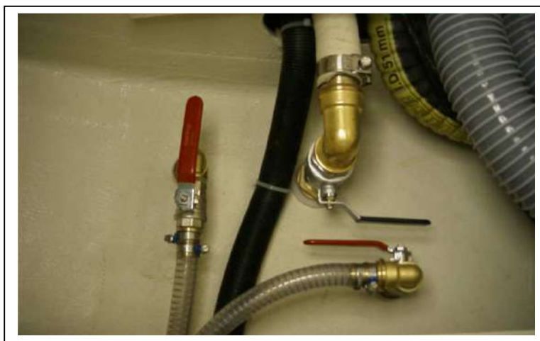
Figure 23: Rapid shut off valve shower room
