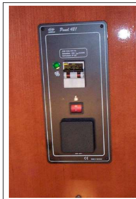
Figure 14: Shore connection panel
